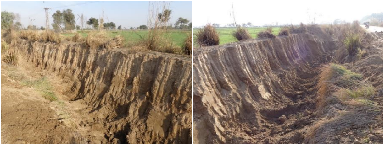
Figure 8. Improper desilting of channels on Joyanwala distributary
